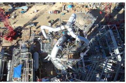
Piping being connected on the top of Stripper Column
